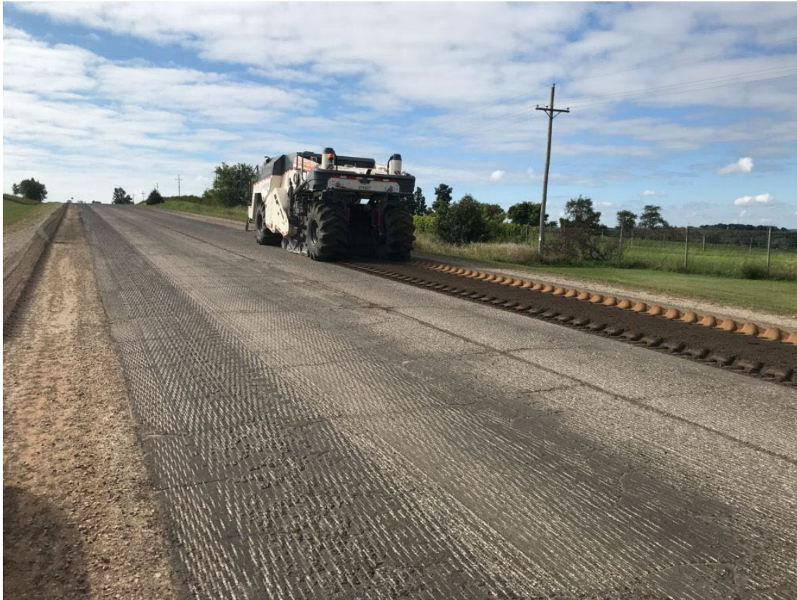
Figure 8: Pulverize and Pave Process Example
