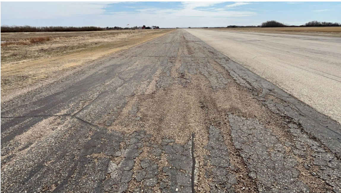
Figure 3: Severely Deteriorated Asphalt on North Edge of Runway
