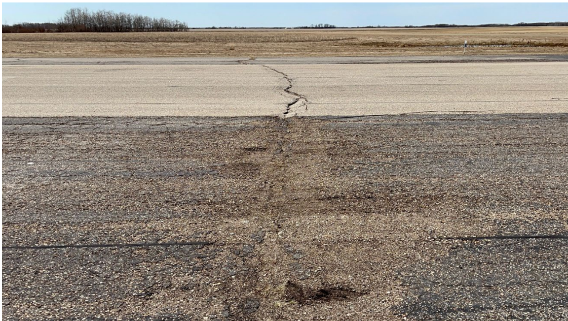
Figure 1: Transverse Crack Example on Runway
