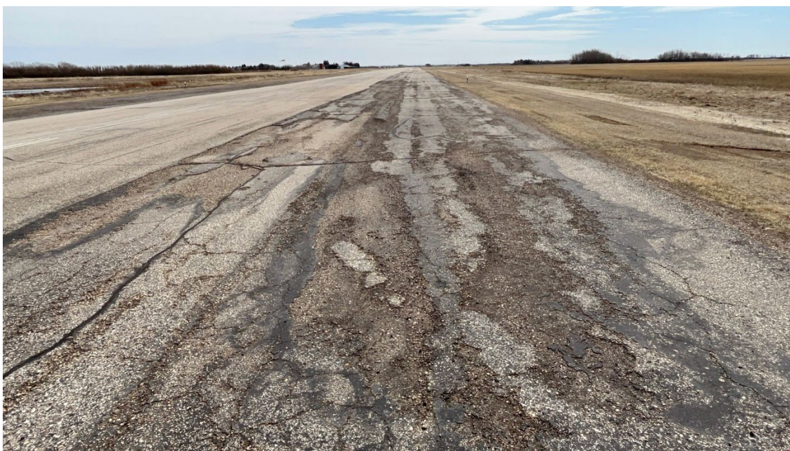
Figure 5: Severely Deteriorated Asphalt on South Edge of Runway
