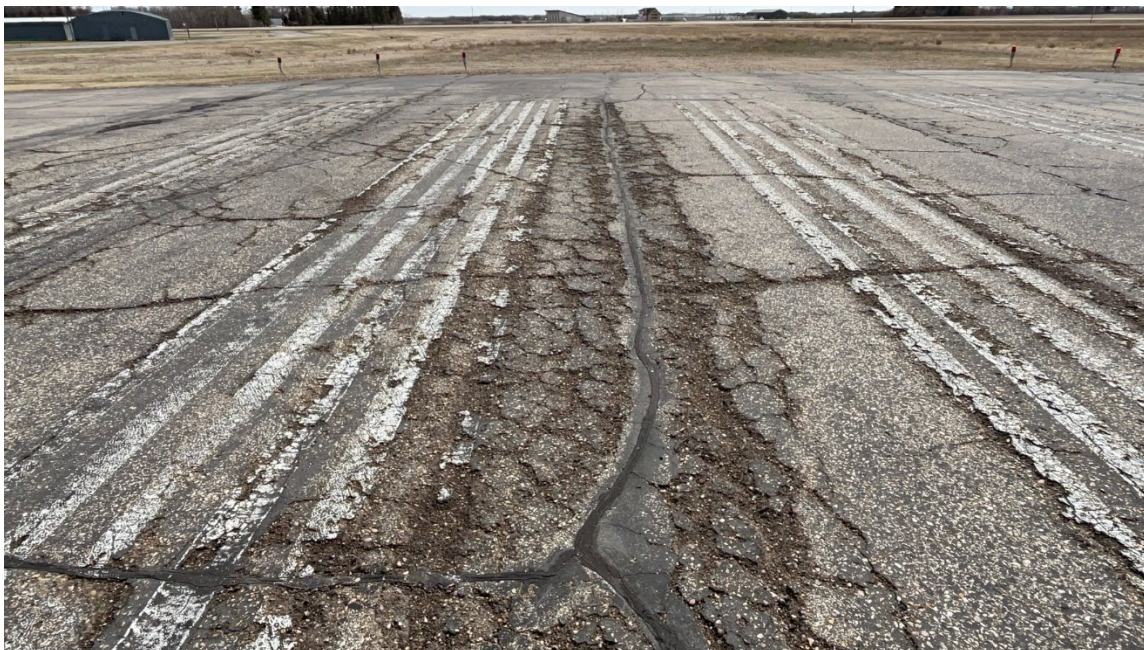
Figure 6: Severely Deteriorated Asphalt at East Threshold (End of Runway)
