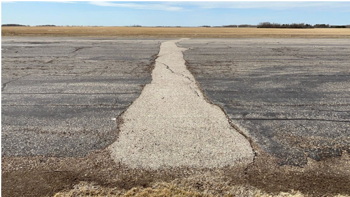
Figure 4: Joint Repair Trial from 2014 - West end of Runway
