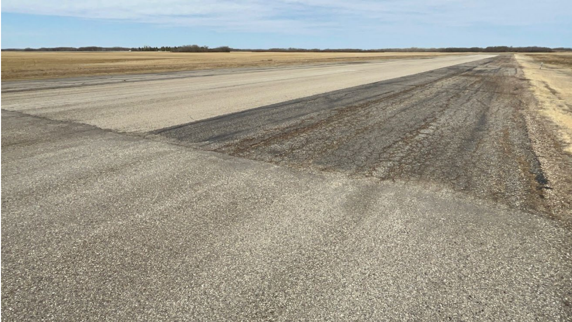
Figure 2: Runway at drainage pipe crossing - Note Different Asphalt Years - 1980's(edges), 2014(centre), 2019(patch)
