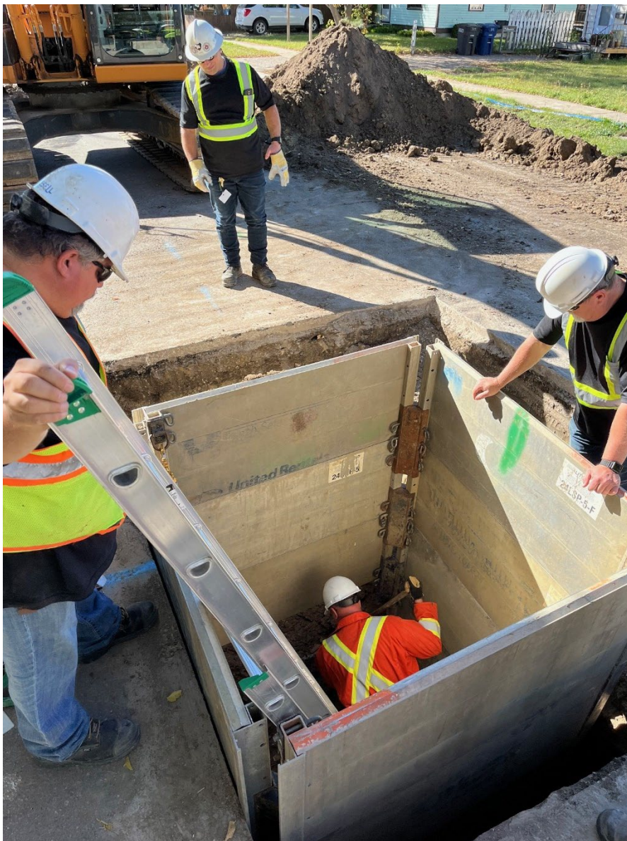
Figure 1: Crews working with Rented Aluminum Trench Shield
