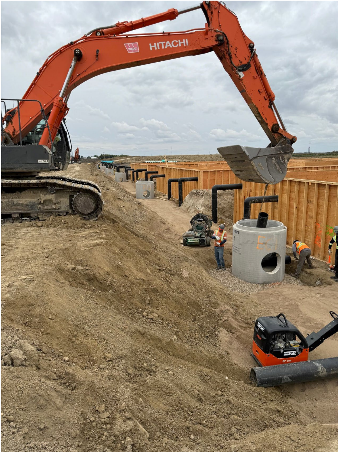
Figure 4: Inlets for the SAGR Cells
