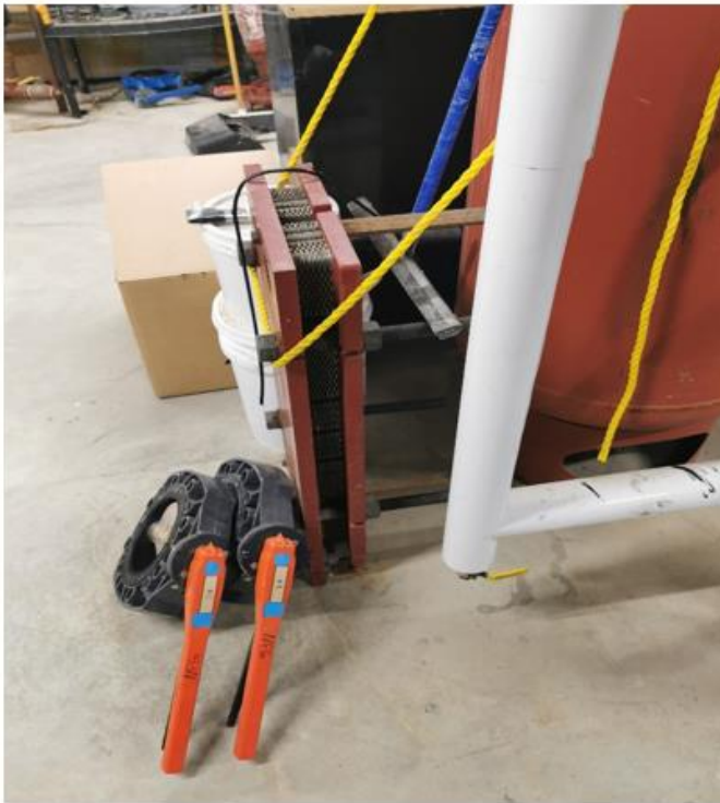
Figure 14: Pool Heat Exchangers
