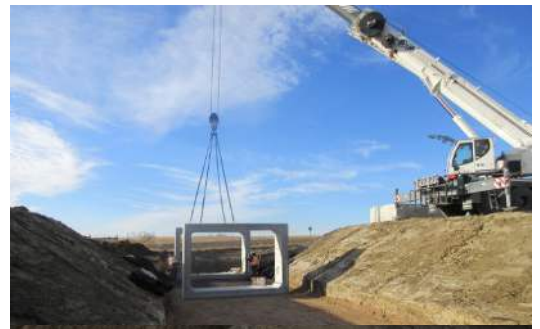
Figure 2: EllisDon installing a box culvert at Mile 9. Courtesy of Howie McInnes
