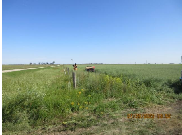
Figure 3: Land Survey Work
