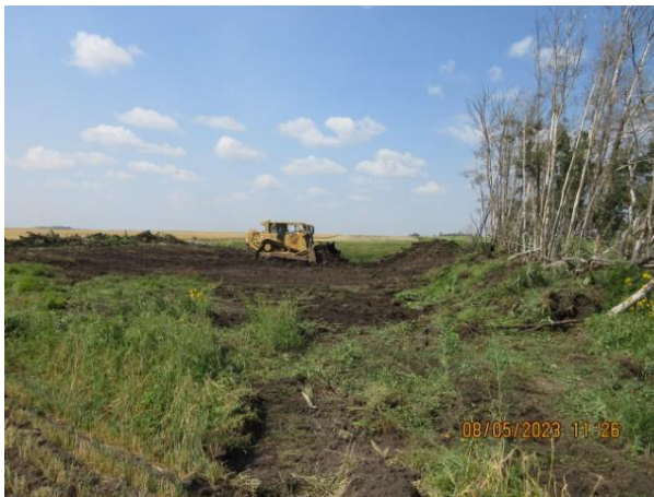
Figure 1: Topsoil Removal
