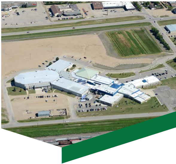
Pictured Above: Humboldt Uniplex 619-17th Street, Humboldt, SK
