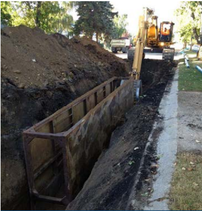
5th Street Watermain Replacement
