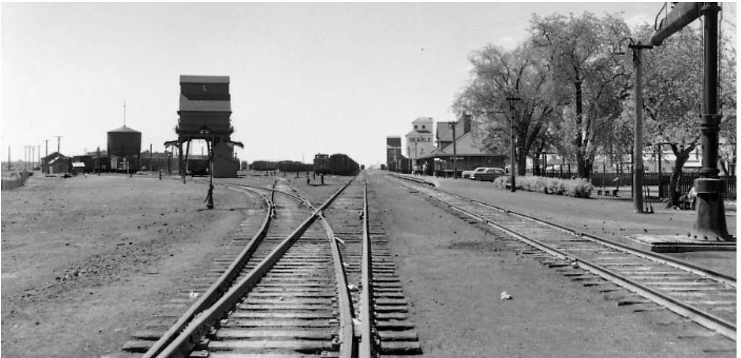
Early 20th Century CN Railway Tracks
