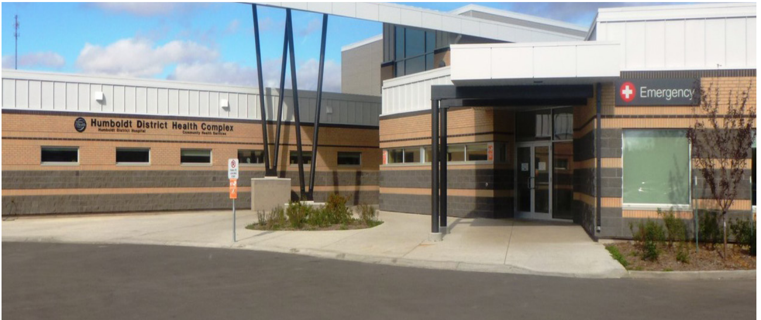
Humboldt District Health Complex
