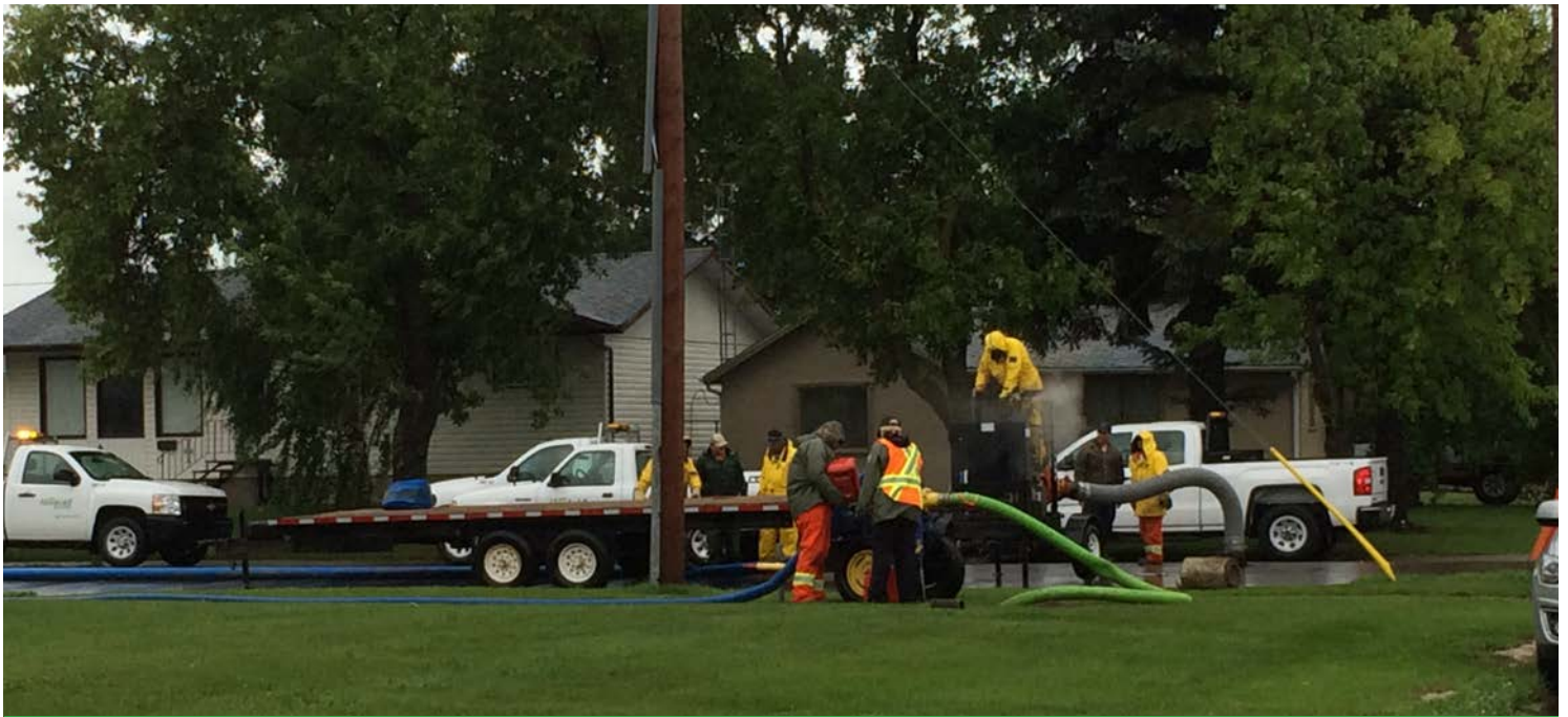
Crews Addressing Storm Sewer Drainage
