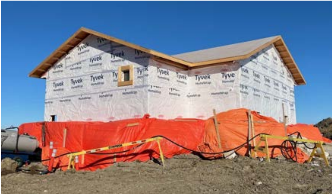
Figure 1: Headworks Building - March 5, 2025
