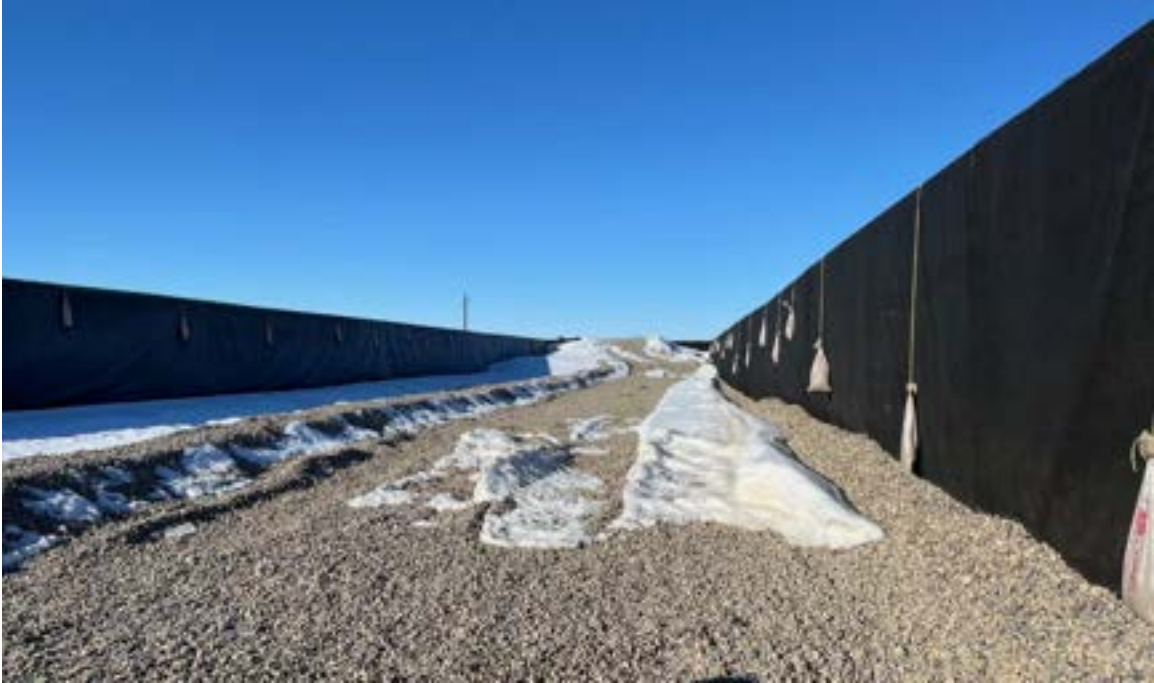
Figure 5: Inside a SAGR Cell - March 5, 2025 – Will be filled with rocks.
