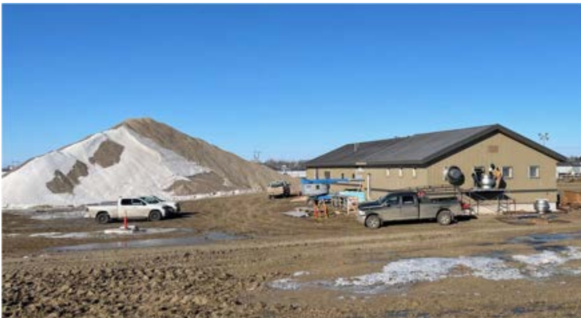
Figure 2: Operations Building, SAGR Rock Pile - March 5, 2025
