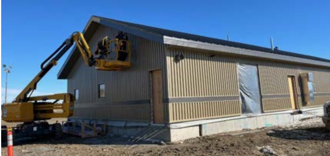
Figure 3: Operations Building - March 5, 2025
